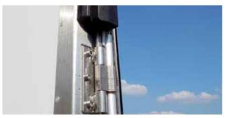
Automatically adjusting double-action spring door hinges
