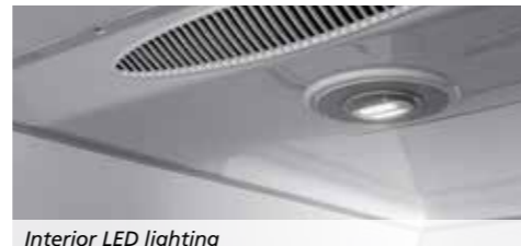
Interior LED lighting
